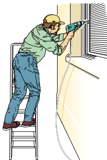
Figure 2a Incorrect - steps side-on to work activity
