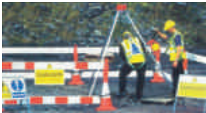
Preparing for a safe confined space entry
